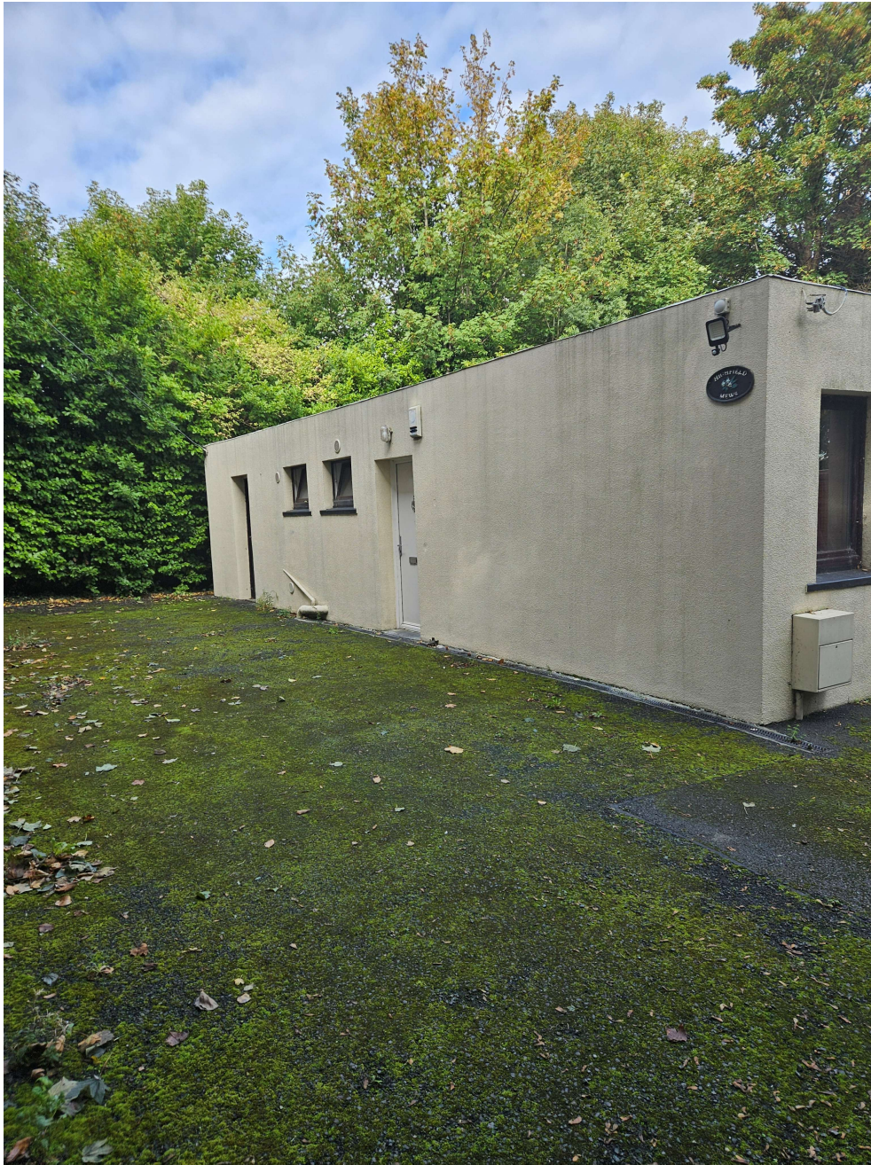
Figure 9: Entrance threshold and external drainage
